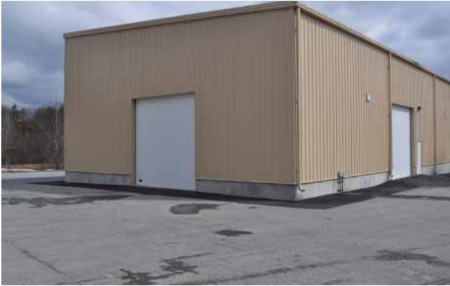
Exterior photo of Landfill Area treatment system
